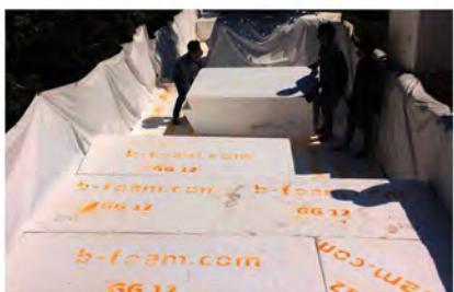
Lightweight Fill, Retaining Wall
